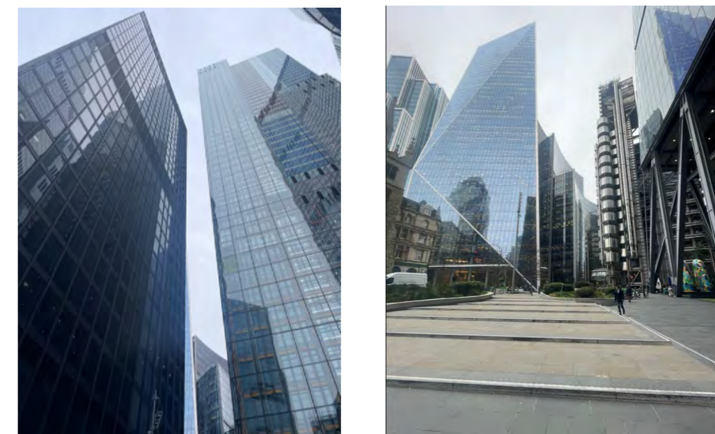
Figure 13 (left): Aviva Tower to the left and rear of the Leadenhall building to the right. Figure 14 (right): View looking south across the square towards 52-54 Lime Street, Lloyds Building to the centre right and Leadenhall Building to the far right. Source: Site images, March 2024 – SLHA.
