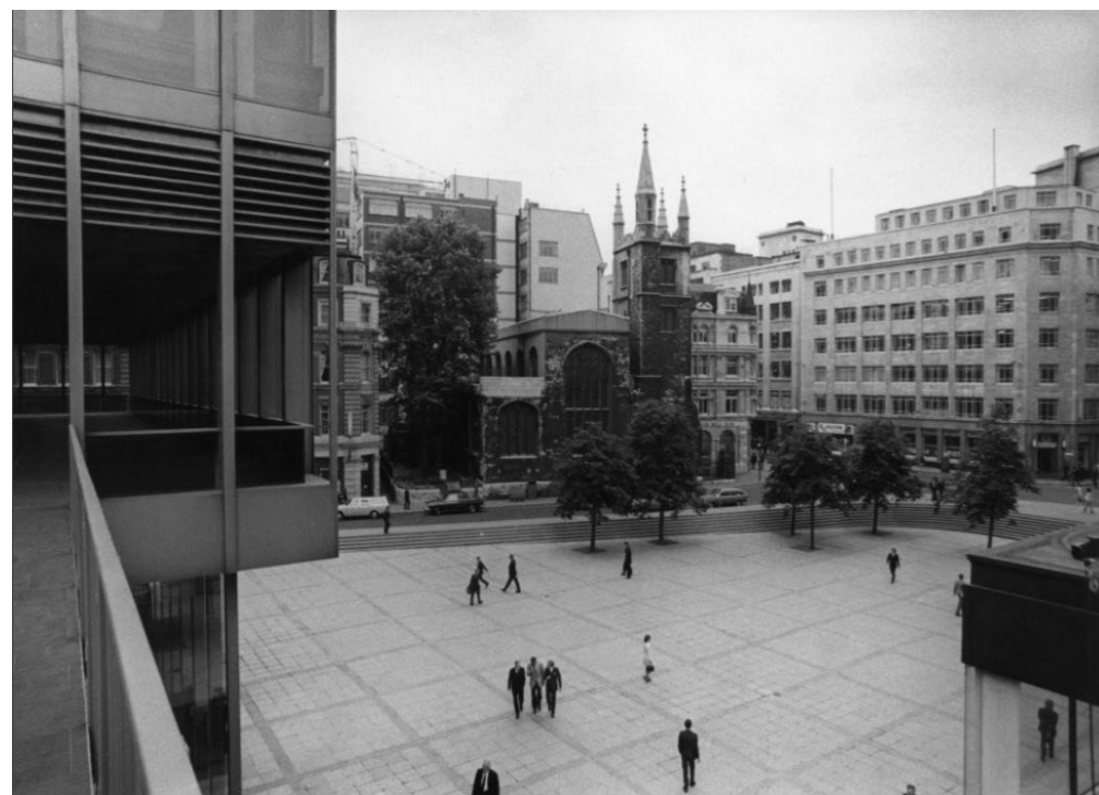
Figure 7: 1973 Commercial Union Tower (Aviva Tower), 1 Undershaft, City of London: the pedestrian walkway leading into the first-floor of the building (podium level), linking to the P&O building. Source: RIBA Ref No RIBA121146.
